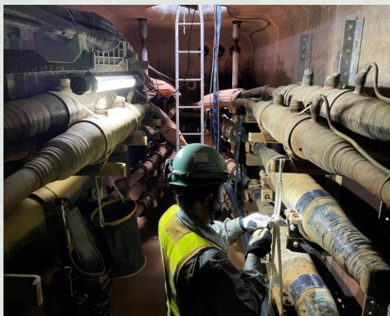
★地中線工事[電気]
